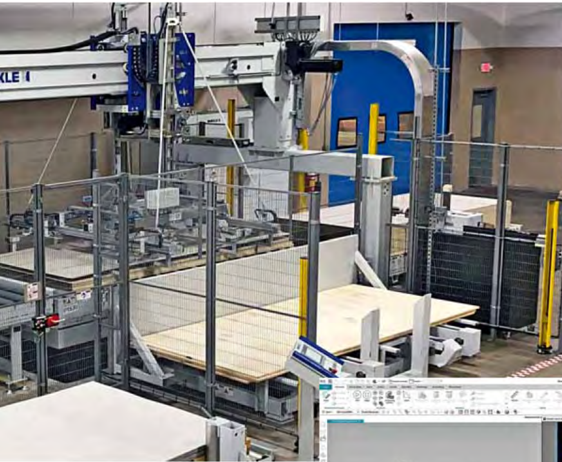
After installation and commissioning. Side view of panel de-stacking with protection board feed (middle) and exit position of the finished stacks (concealed at the rear) with panels passing through
